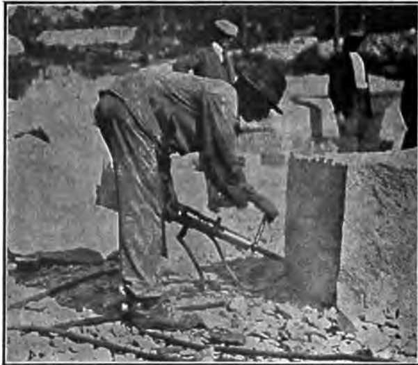
Fig. 117. Plug Hole Drilling.
